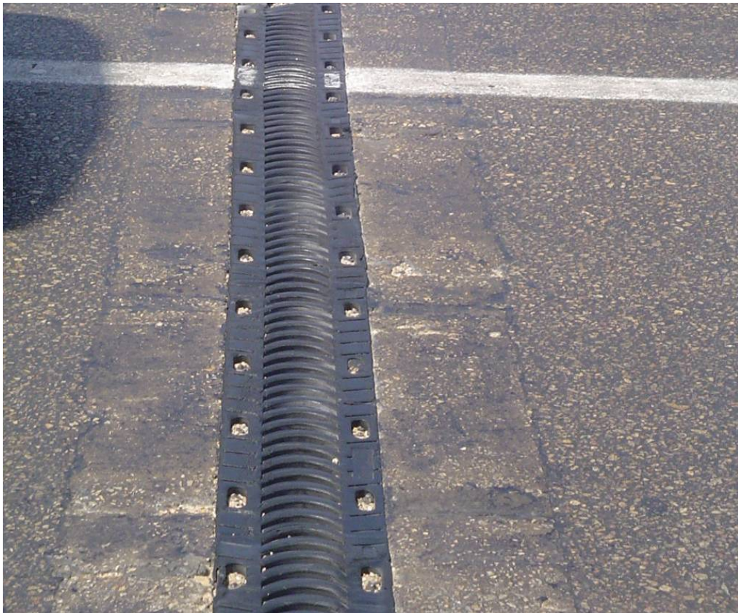
Figure (3-9) Closed 'sealed' bridge joint.
