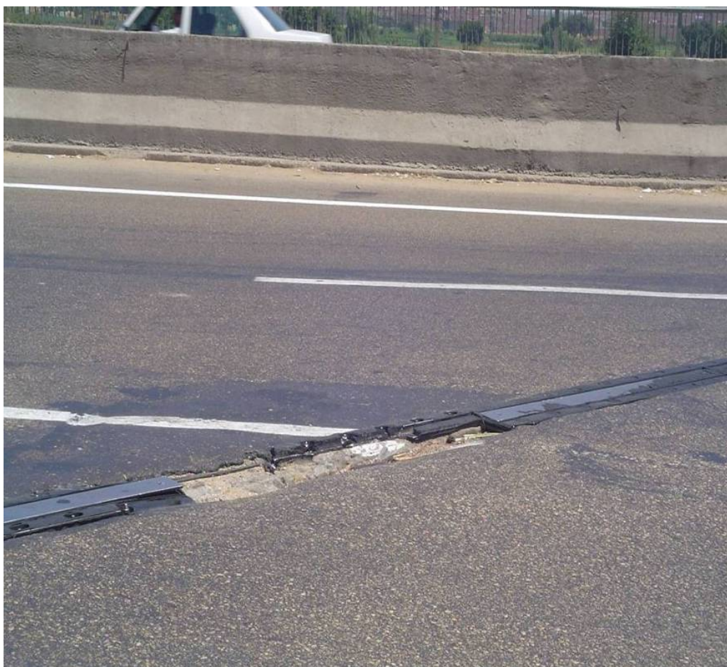
Figure (3-11): Damaged bridge joint, inner carriageway, (km 67.3).
