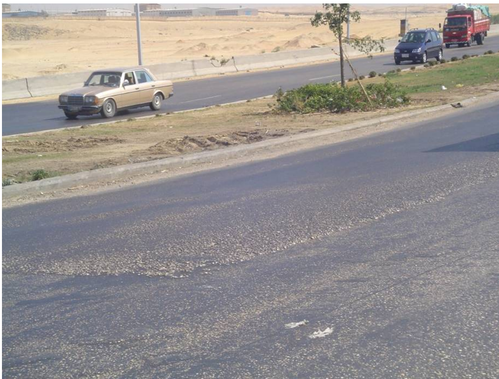
Figure (3-3): Depression and corrugation, outer carriageway, (km 23).
