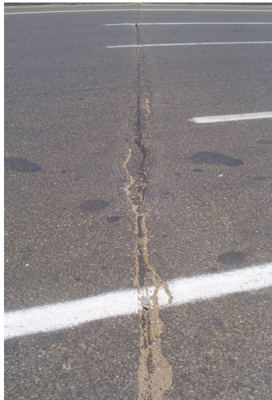
Figure (3-7): Transverse crack, inner carriageway, (km 69.9).
