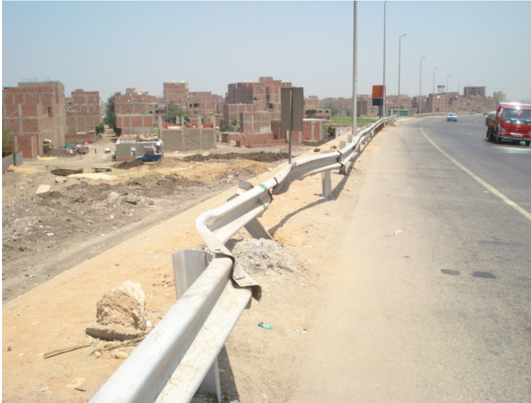
Figure (3-13): Damaged W-beam traffic guardrail, outer carriageway, (km 88.5).
