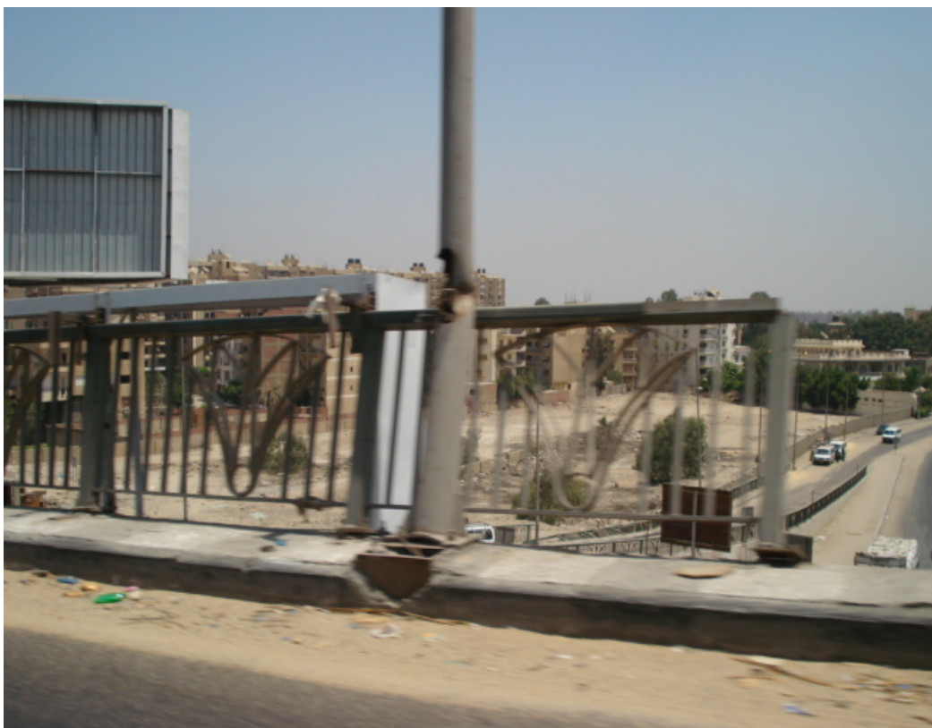
Figure (3-15): Damaged bridge rail, inner carriageway, (km 90.9).
