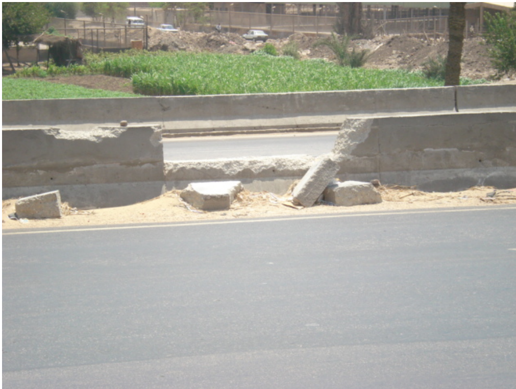
Figure (3-14): Damaged median concrete barrier, (km 88.5).
