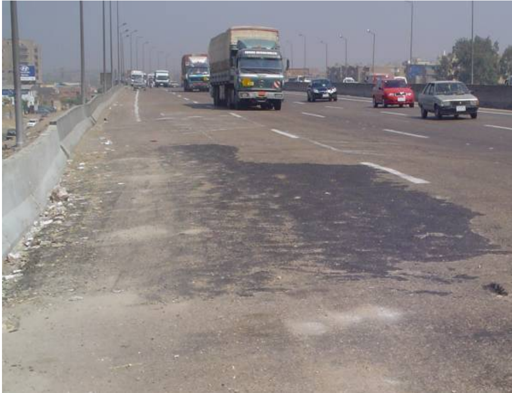
Figure (3-6): Bleeding, inner carriageway, (km 49.4).
