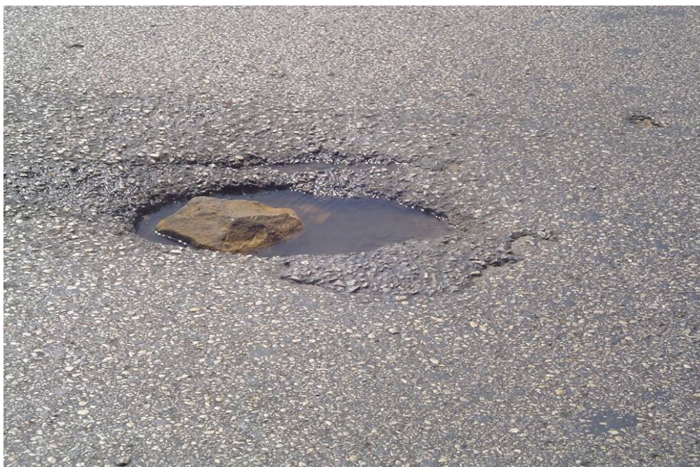
Figure (3-4): Pothole, outer carriageway, (km 23.5).
