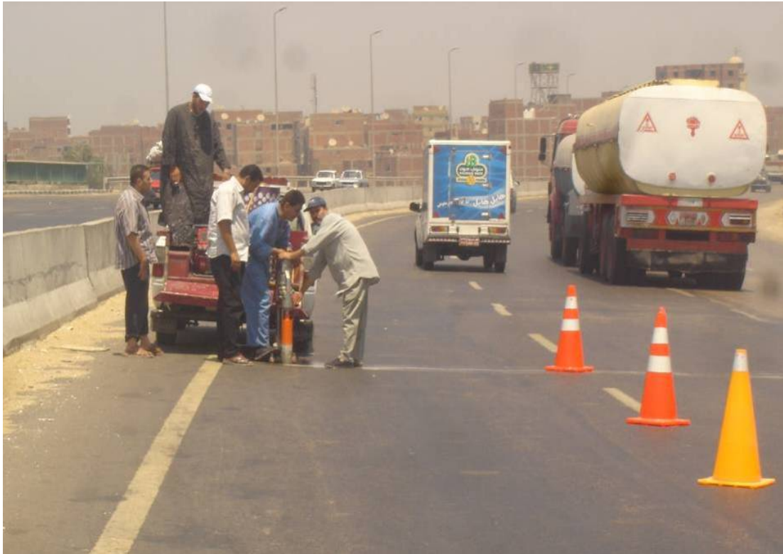
Figure (4-3): Sample of core extraction.
