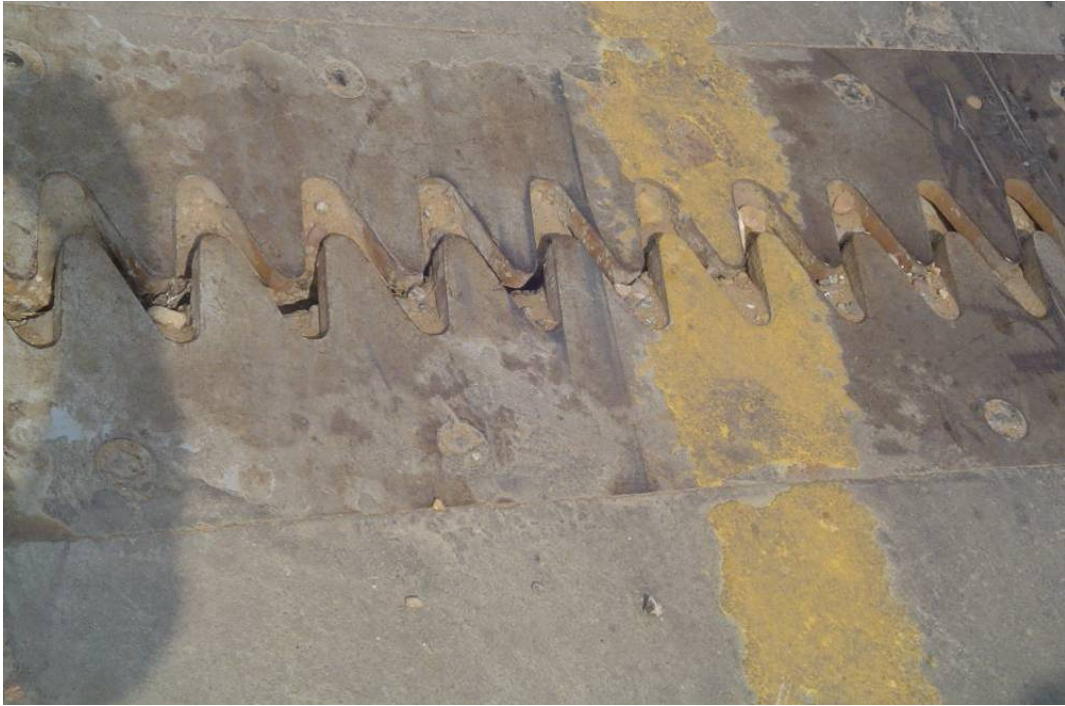
Figure (3-8): Bridge finger joint.
