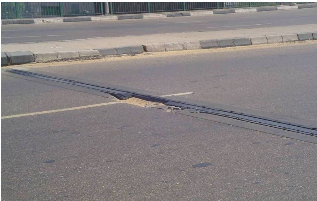
Figure (3-10): Damaged bridge joint, outer carriageway, (km 7.2).
